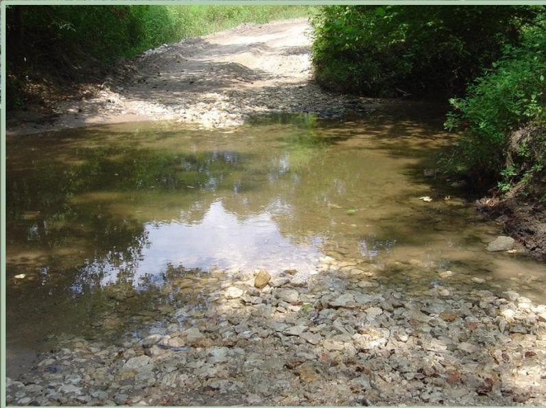
A permanent crossing for low flow streams with low banks and a firm stream bed suitable for driving across
