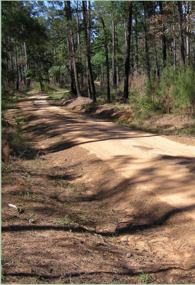
Road in which the centerline is the highest point on the road plane
