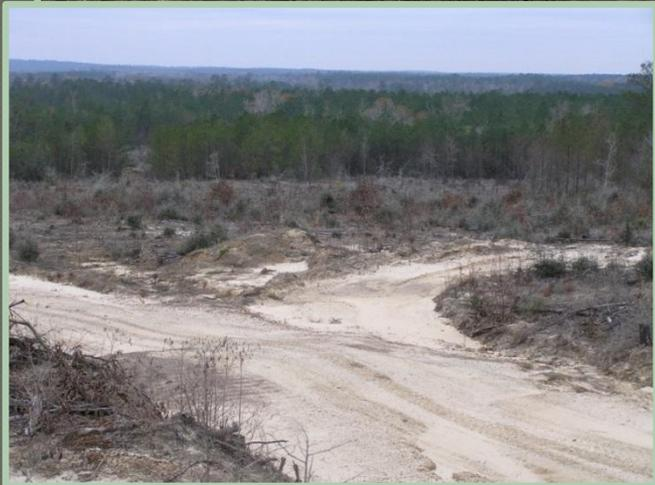
A water turnout or diversion ditch constructed to move and disperse water away from the road.
