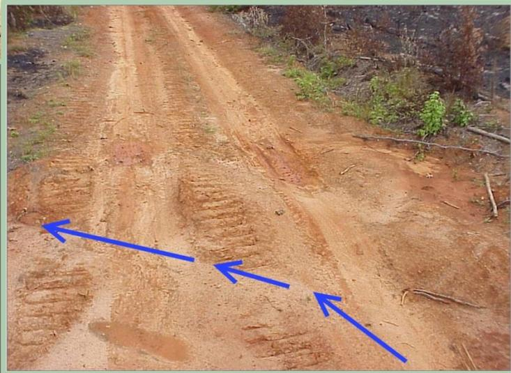
A cross drainage diversion ditch and/or a hump in a trail or road for the purpose of diverting surface water runoff into roadside vegetation
