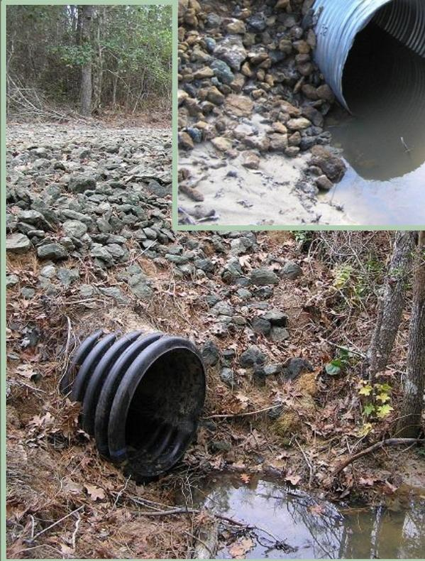
A conduit or pipe through which surface water can flow under roads that cross streams
