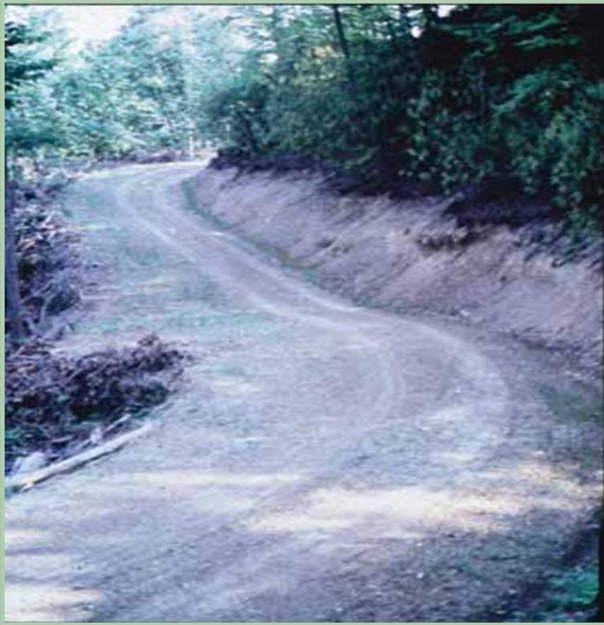
A shallow depression built diagonally across a light duty road or trail to divert surface water runoff from the road or trail.
