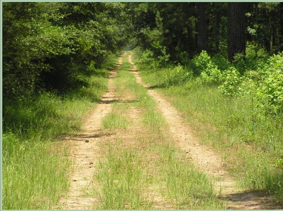
Removal of trees along the edges of a road to reduce the shade and promote faster drying of the road surface.
